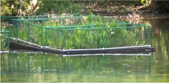
In summary, septic waste of the community will be collected through main pipes and delivered to the communal septic tank and from there it will undergo the first treatment. After that, the treated wastewater would be discharged into the river. When it is already in the river, it will undergo the second treatment which is the Floating Wetland. Water quality of the river will be improved with this proposed solution.
